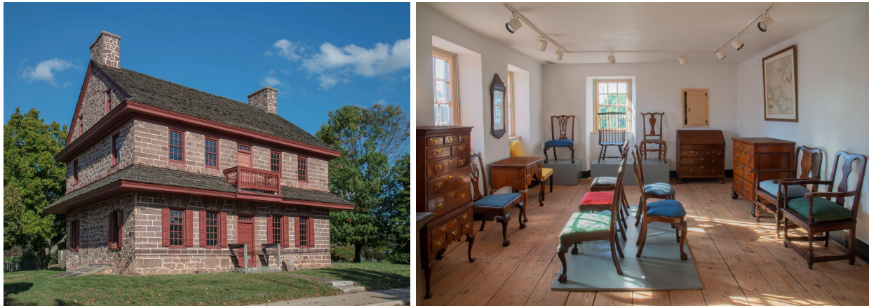
The Henry Muhlenberg House exterior and furniture gallery. Courtesy of Historic Trappe, photos by Gavin Ashworth.
